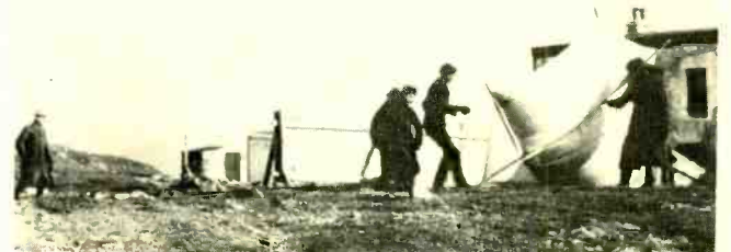
MARCONI (extreme left) and assistants launch kite that raised antenna used at Signal Hill, Newfoundland to receive the first wireless signals from across the Atlantic Ocean. Storm made reception very difficult.
