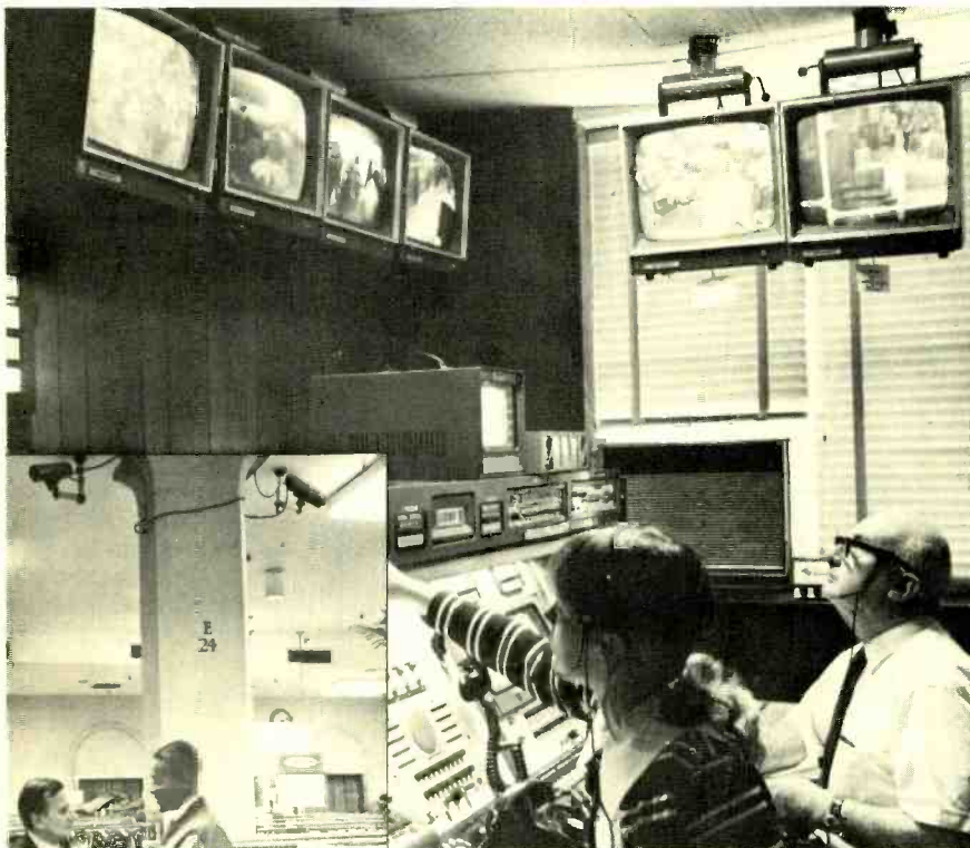
CONTROL CENTER AT MACY'S Herald Square store. Dispatchers sit before radio console and CCTV monitors. Here, they can reach or observe personnel throughout the 21 floors of the store. Center is focal point of the radio system and controls a combination of approximately 50 small 2-way radios and pocket pagers used by security personnel throughout the store. Two smaller monitors for close-ups (inset) are in the console.
